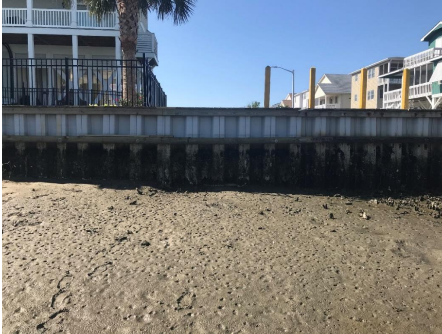
Figure 4. Existing Vinyl Sheetpile Wall (Cobia Street)
